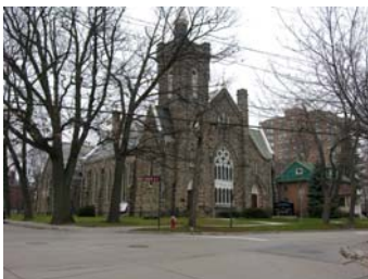
St Andrews Presbyterian - Church Street
