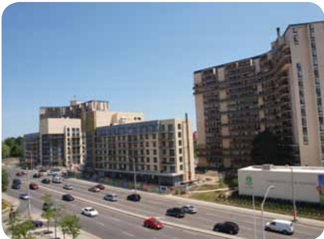
New street related construction in front of existing apartment buildings, Shepard Avenue, Toronto
