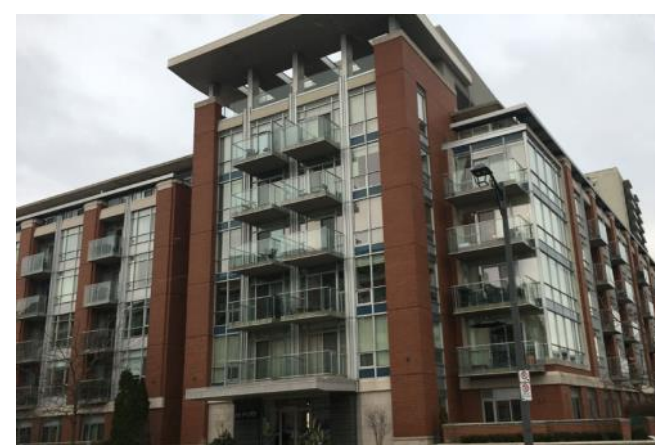
Residential Third Density - Mid Rise (R3M): Provides for mid-rise apartments up to 12 storeys
