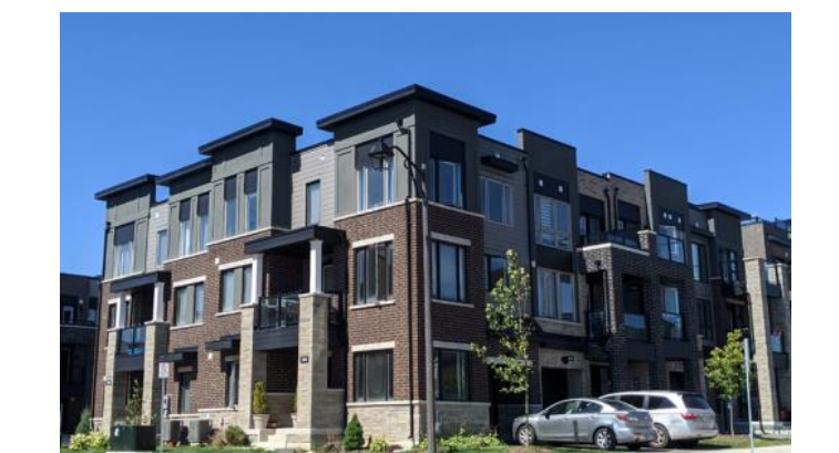
Residential Second Density Type A (R2A): Provides for multiple townhouse units such as stacked and back-to-back townhouses
