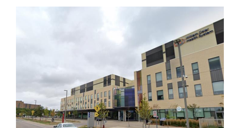
Major Institutional (I2): Major Institutional provides for large-scale institutional uses such as hospitals and post-secondary education uses
