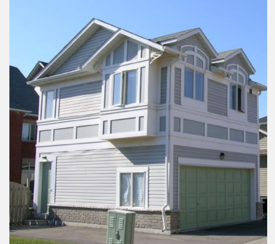
Example of a coach house ARU above a detached garage on a rear lane
