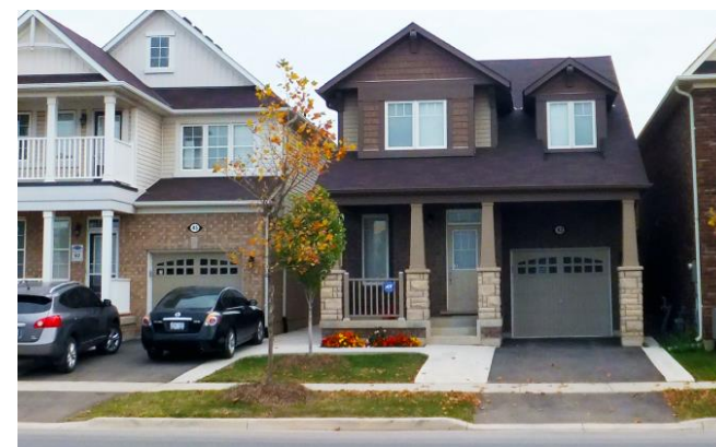
Residential First Density (R1): Provides for single detached houses, semi-detached houses + up to two additional residential units (ARUs) on a variety of lot sizes
