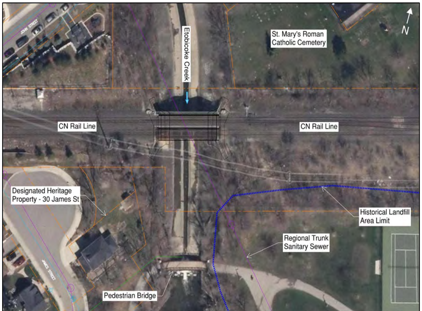
Figure 2 CN Crossing of Etobicoke Creek – Existing Condition
