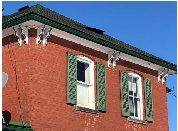
Plate 20: Typical windows and paired wooden brackets.
