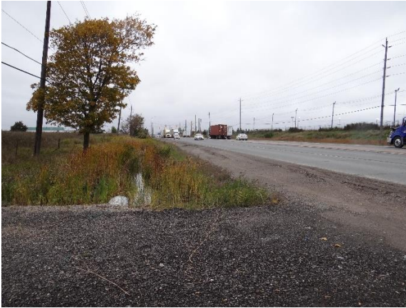
Plate 1: View of Highway 50, looking northwest, adjacent to the study area.
