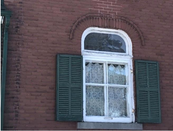
Plate 21: First-storey window with leaded-glass transom and projecting brick arch on east elevation.
