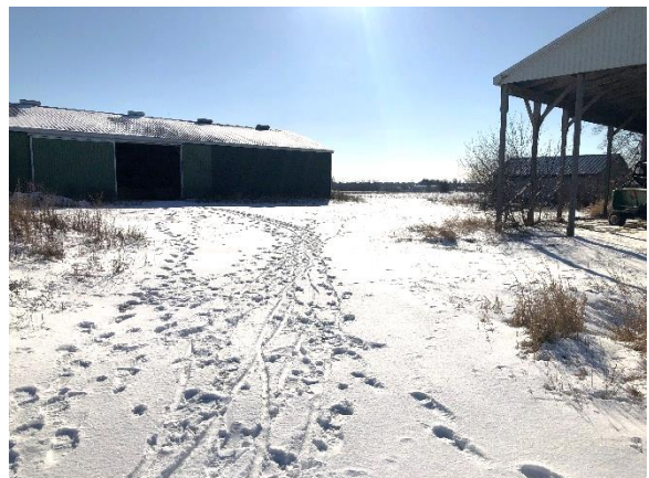
Plate 35: Looking south towards aluminum-clad building.
