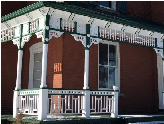
Plate 25: Detail of verandah woodwork.
