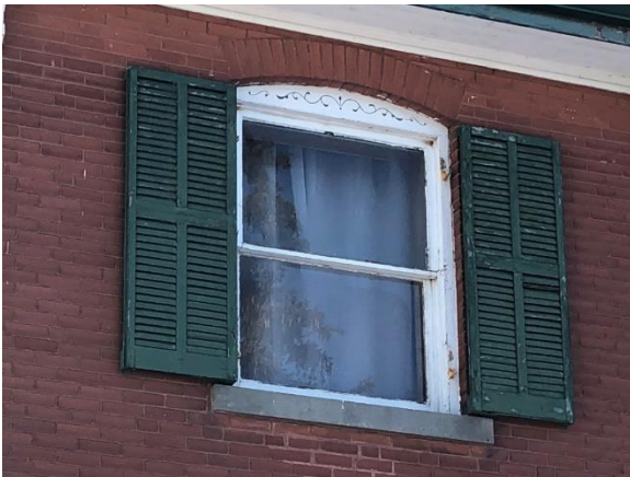
Plate 23: Second-storey window with decorative carved head on east elevation.
