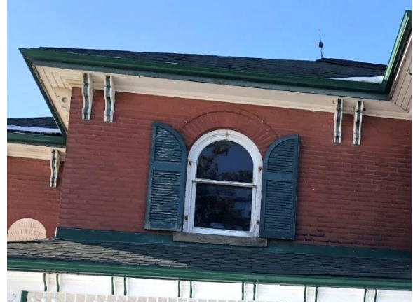
Plate 22: Second-storey window with semi-circular arched head and projecting brick arch.
