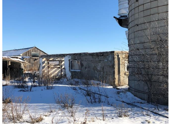
Plate 31: Looking east towards concrete barn foundation.
