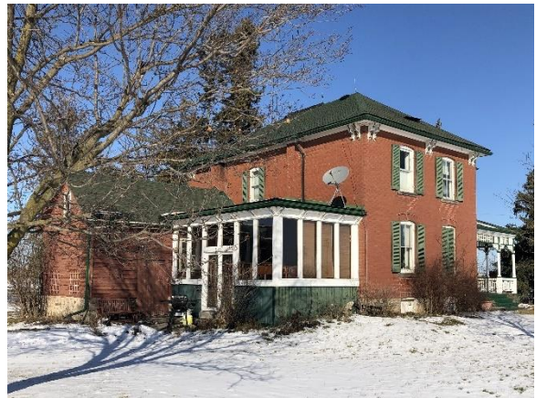
Plate 18: West and south elevations of the house with one-storey tail and enclosed porch.
