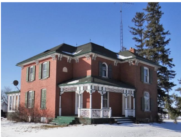
Plate 13: South and east elevations of the house.
