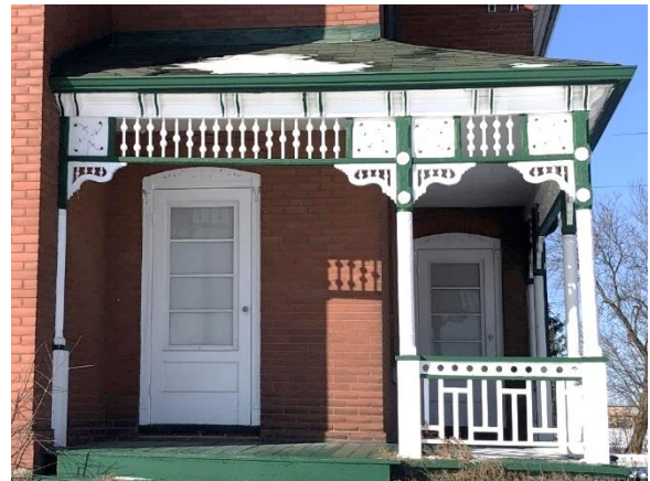
Plate 24: Matching entryways on south elevation.
