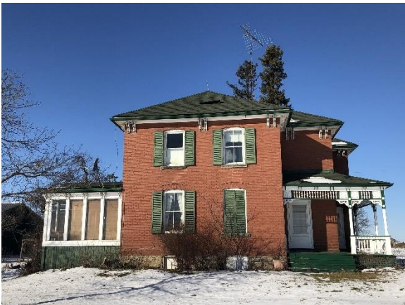
Plate 19: South elevation of the house.
