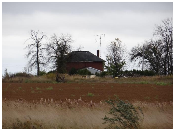
Plate 8: Rear of the property located at 10307 Clarkway Drive, looking west.
