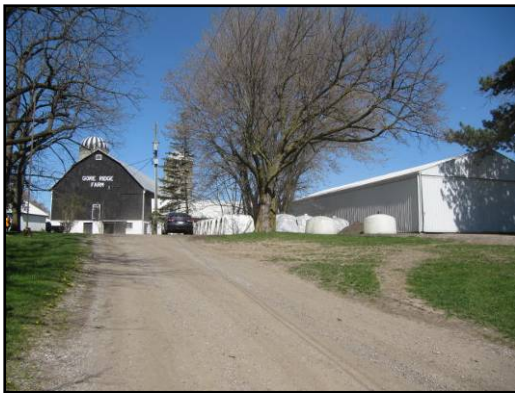
Plate 7: Looking northeast towards farm complex and gravel driveway
