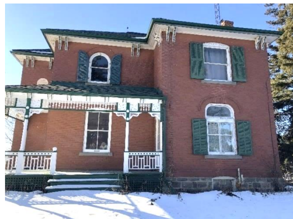
Plate 14: East elevation of the house.
