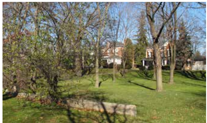
Remaining retaining wall at 56 and 58 Main Street South (Source: ERA).
