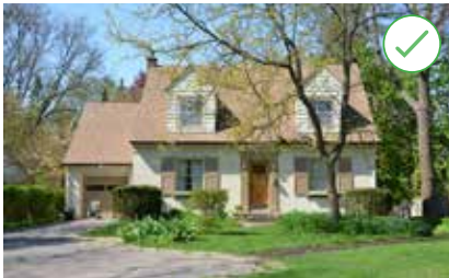
This attached garage is set back from the front façade and uses corresponding materials and roofline which maintain the character and prominence of the dwelling (Source: City of Brampton)
