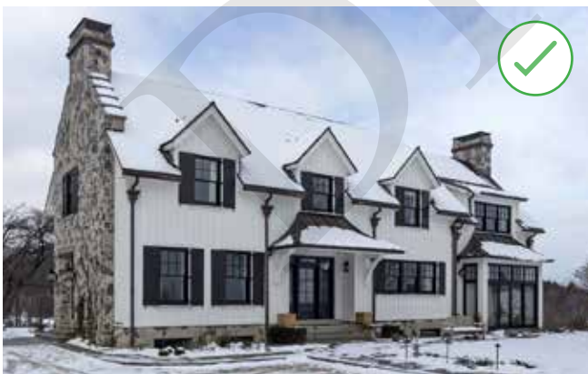
This modern farmhouse in the outskirts of Collingwood is a contemporary design, but blends with the area's rural character and employs traditional farmhouse design methods in responding to the region's rugged landscape. (Source: ERA Architects, Vik Pahwa)
