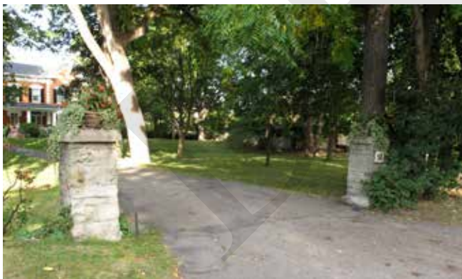
Remaining bridge piers at 58 Main Street South (Source: ERA).
