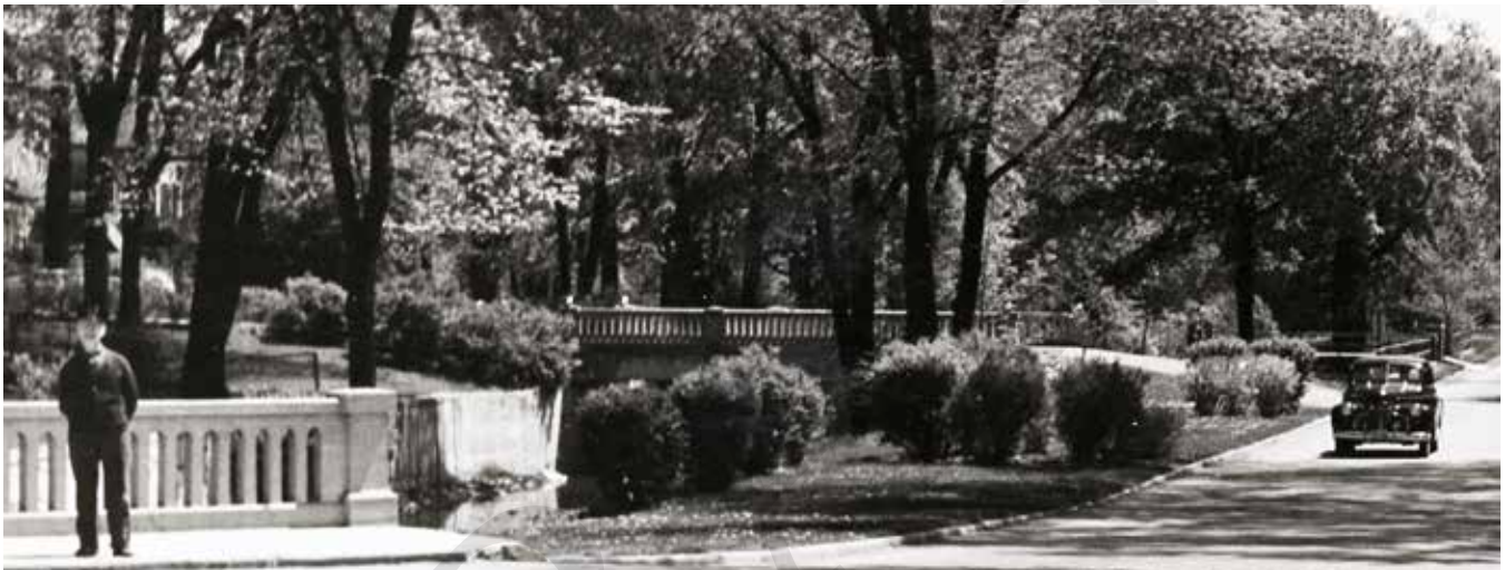
Historic photograph of the driveway bridge from the street to 58 Main Street South (Source: PAMA).
