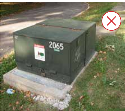
Installation of public utilities on Main Street South impacts the heritage character of the streetscape. (Source: ERA)
