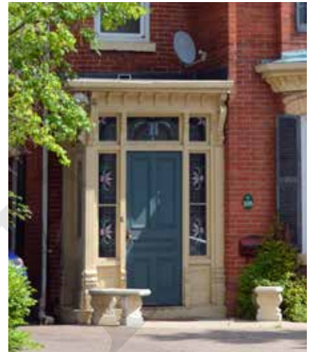
The door, surround, and transom and sidelights on the entrance at 108 Main Street South all help to convey the residence's Italianate architectural style (Source: ERA)
