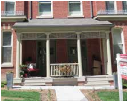
Porch conservation using an archival photograph to understand the original condition. Images show the historic condition (top), the recent deteriorated condition (middle), and the reinstated porch (bottom). (Source: ERA)
