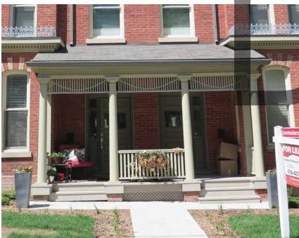
Porch conservation using an archival photograph to understand the original condition. Images show the historic condition (top), the recent deteriorated condition (middle), and the reinstated porch (bottom). (Source: ERA)
