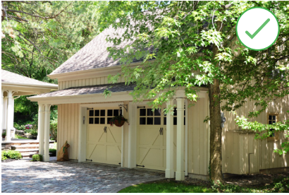
This detached garage addition is set back and also complements the design of the historic dwelling on the property (Source: City of Brampton)
