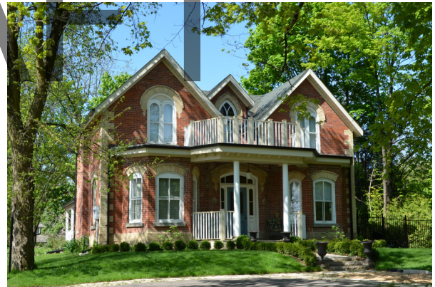
Buildings in the District represent a rich diversity of architectural styles, including 133 Main Street South’s Gothic Revival style (Source: ERA)
