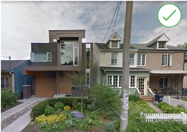
Despite being taller than its contributing neighbour, this new construction in a Toronto HCD clearly responds to its neighbour's height through the primary façade's roofline, and sets back its higher section so that it appears subordinate (Source: Google Streetview, 2014)
