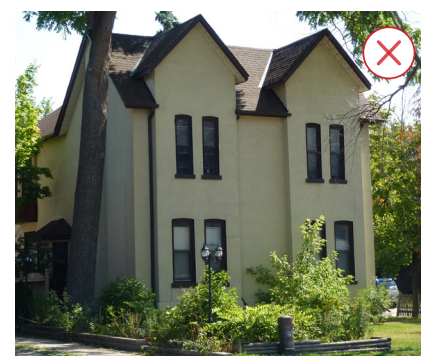
This house illustrates the application of new cladding material over historic brick, which detracts from the character of the building and conceals architectural details. (Source: ERA)
