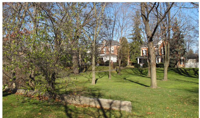
Remaining retaining wall. (Source: ERA)
