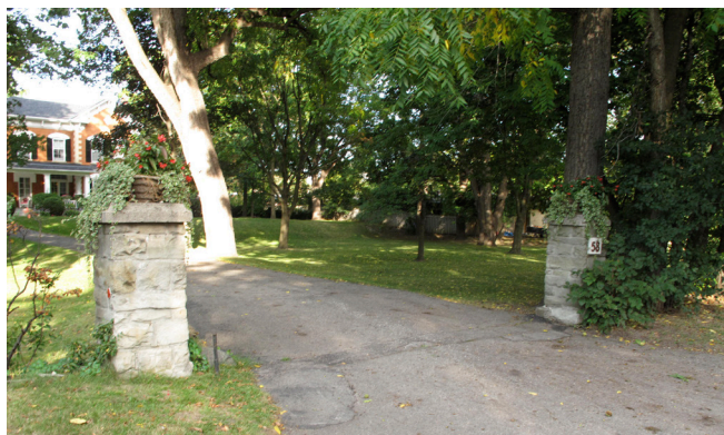
Remaining bridge piers. (Source: ERA)
