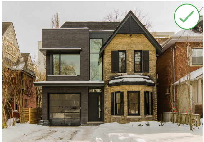
This addition picks up linear design cues from the historic residence, and speaks to its window openings, colour tones and materiality while presenting as modern architecture (Source: Larendale Group)
